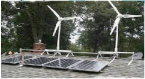
Solar-PV Wind hybrid power specifications are given below PV Array Power = 20 watts Wind turbine/generator = 3 W
